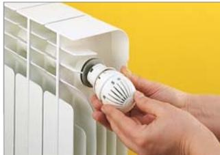
2. Fasten the thermostatic head to the valve aligning the half moon shaped gaps at the base of the head with the protruding lugs on the valve.
