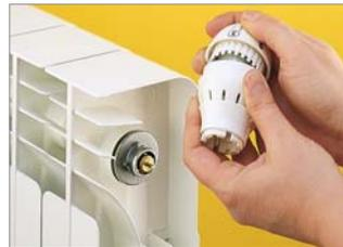
1. Turn the handle to the desired setting position and take it off by pulling it forward. Do not tamper with the position of the thermostatic sensor for any reason, not to lose the calibration of the thermostatic head.
