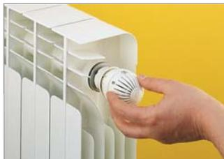
3. Close the head completely turning to this position
